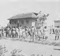
A CROWD of interested spectators was on hand, above, to see the first section of the building reach its new site. In the background, below, is the St. Ana Church at Noord.
